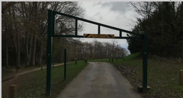
Figure 2 – Vehicle height restriction at entrance road to Lower East Court play area car park
